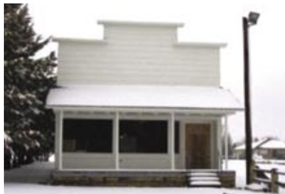
Undergoing restoration - winter 2005
